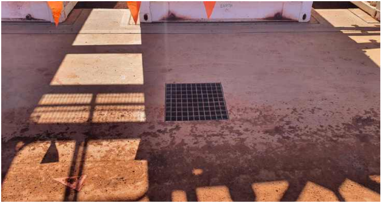
Photo 5 Spillage sump
