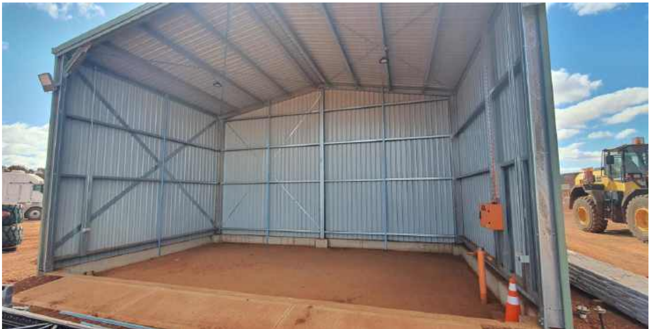
Photo 6 Reagents shed with bunding
