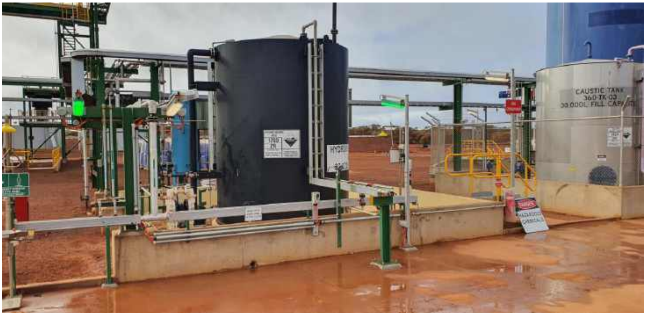
Photo 2 Hydrochloric acid tank bunding
