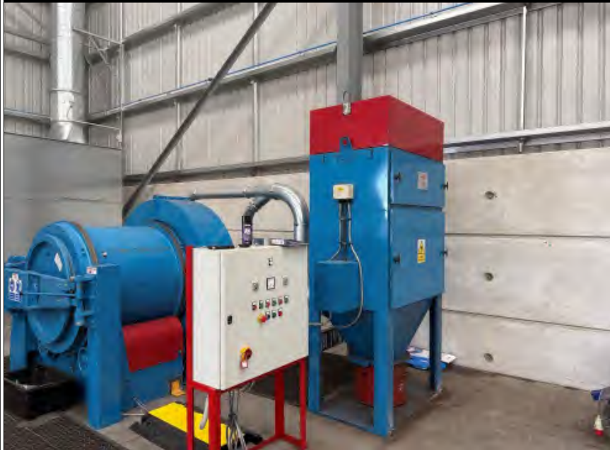
SHOT BLASTING CHAMBER AND DUST EXTRACTION SYSTEM
