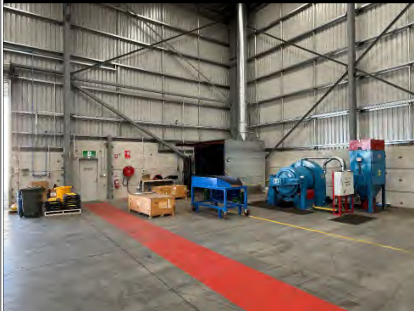
INTERNAL VIEW – PLASMA-CUTTING AND ABRASIVE CLEANING AREA
