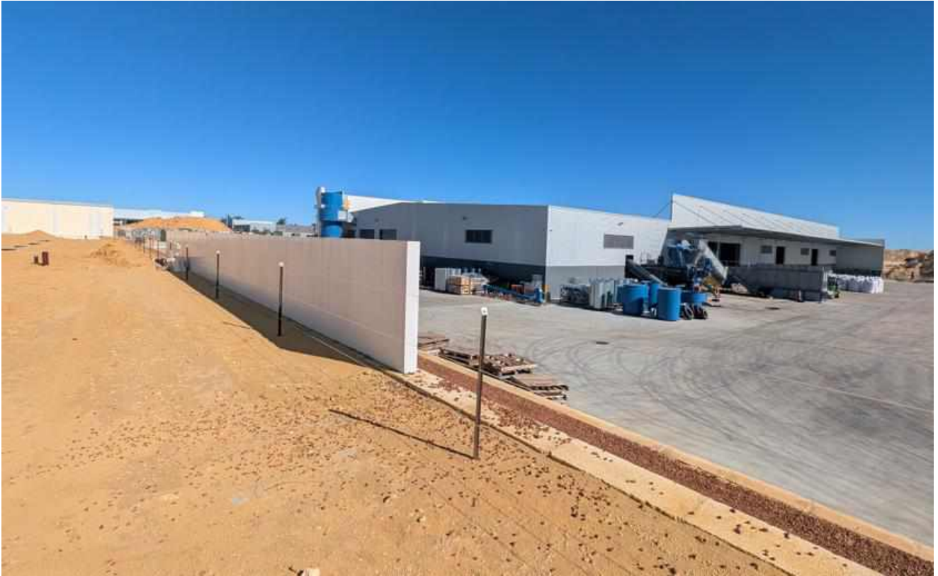
Figure 3-3 Partially Completed Noise Wall
