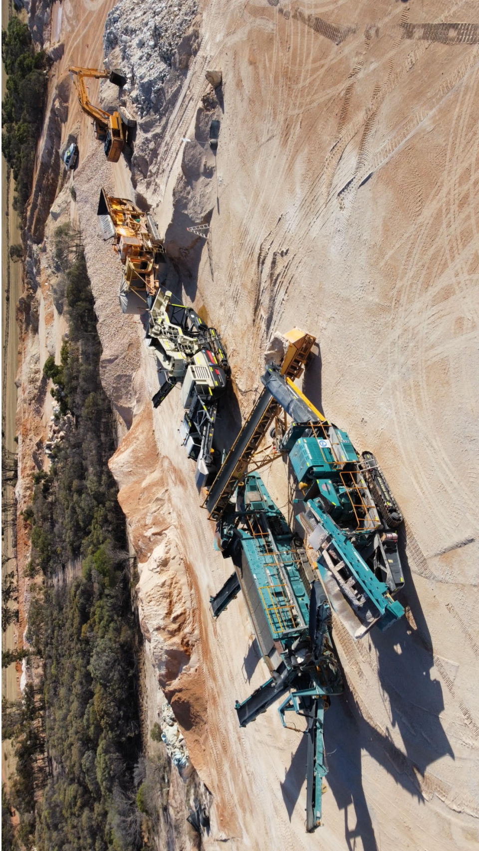
Typical Mobile Site Arrangement (photo of existing operation at nearby location)
