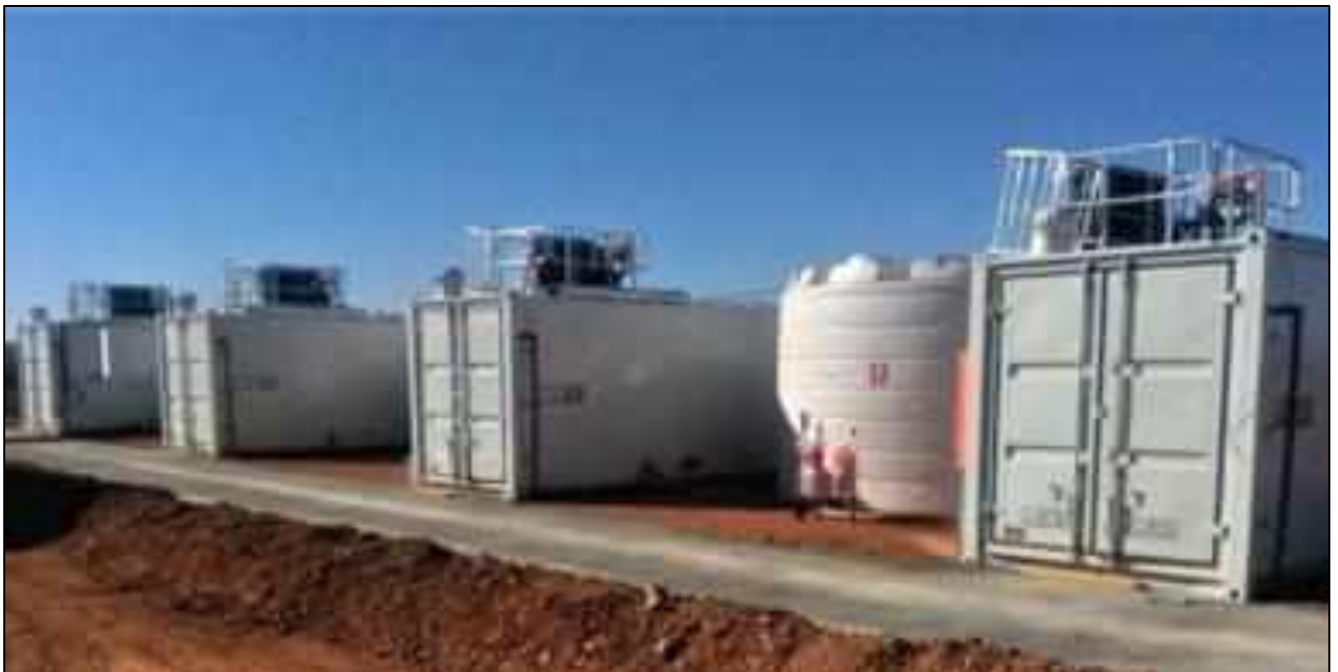
Figure 2.6 Example SBR WWTP (4 x process trains)
