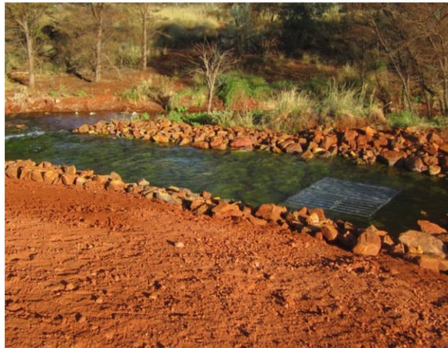
Figure 13: Example of an ‘upwelling’ type discharge outlet at Yandicoogina DO6 (RTIO, March 2017a)
