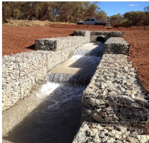
Figure 11: Example of a ‘gabion-style drop structure’ type discharge outlet at Yandicoogina DO9 (RTIO, March 2017a)
