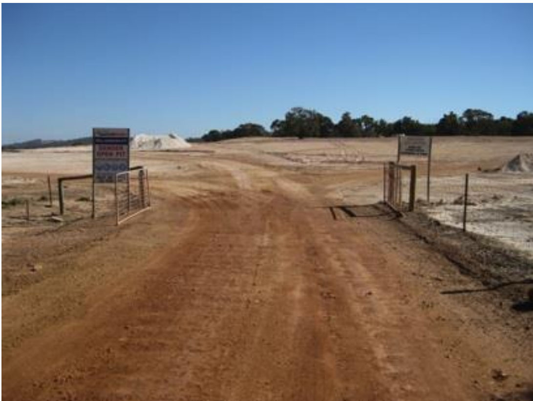
View of Clay Pit Entrance
