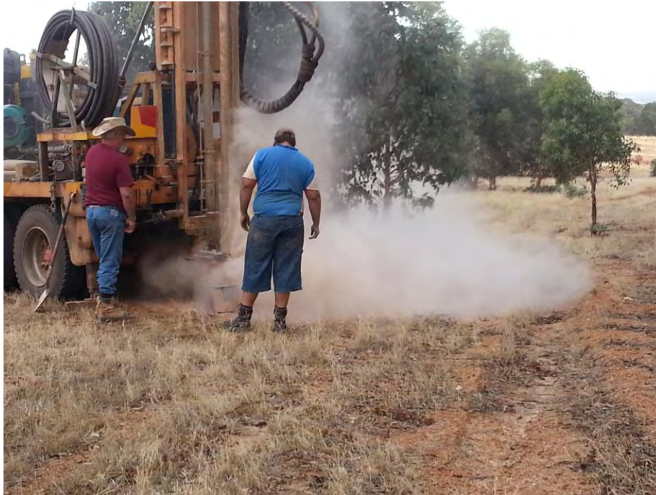
Drilling at depth showing dry conditions
