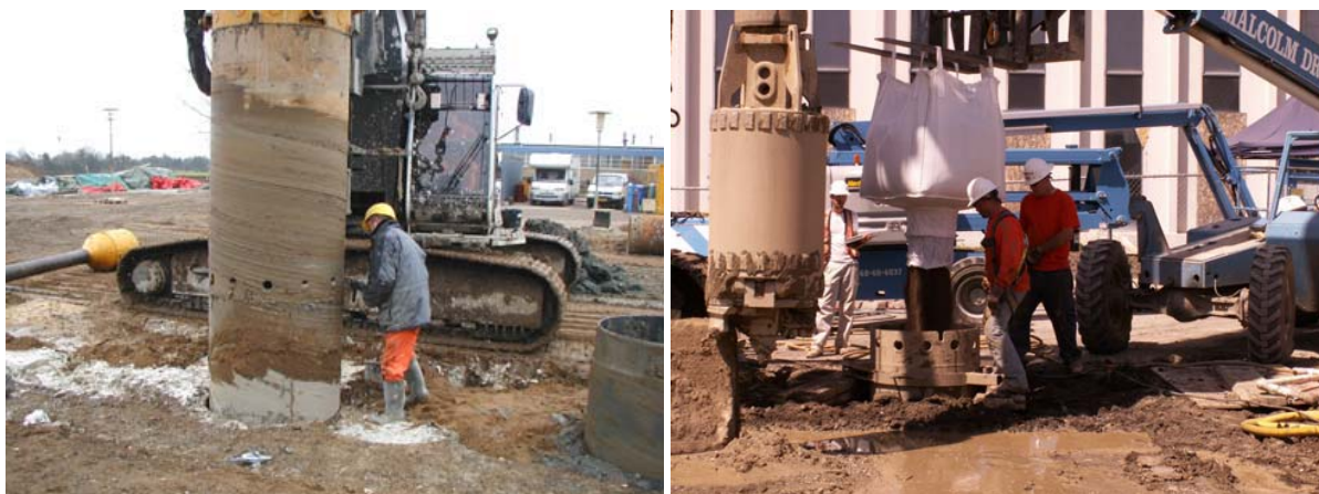
Figure B: Photos showing PRB construction with secant caisson and filling of caisson with ZVI/sand mixture- courtesy of ETI.
