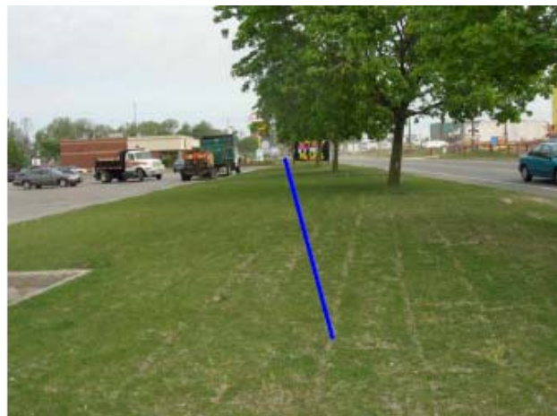
Figure G: Photos showing reinstated ground conditions approximately one year after PRB installation in Cambridge, Canada. Blue line shows approximate location of PRB. Note monitoring point in the foreground of left photo.
