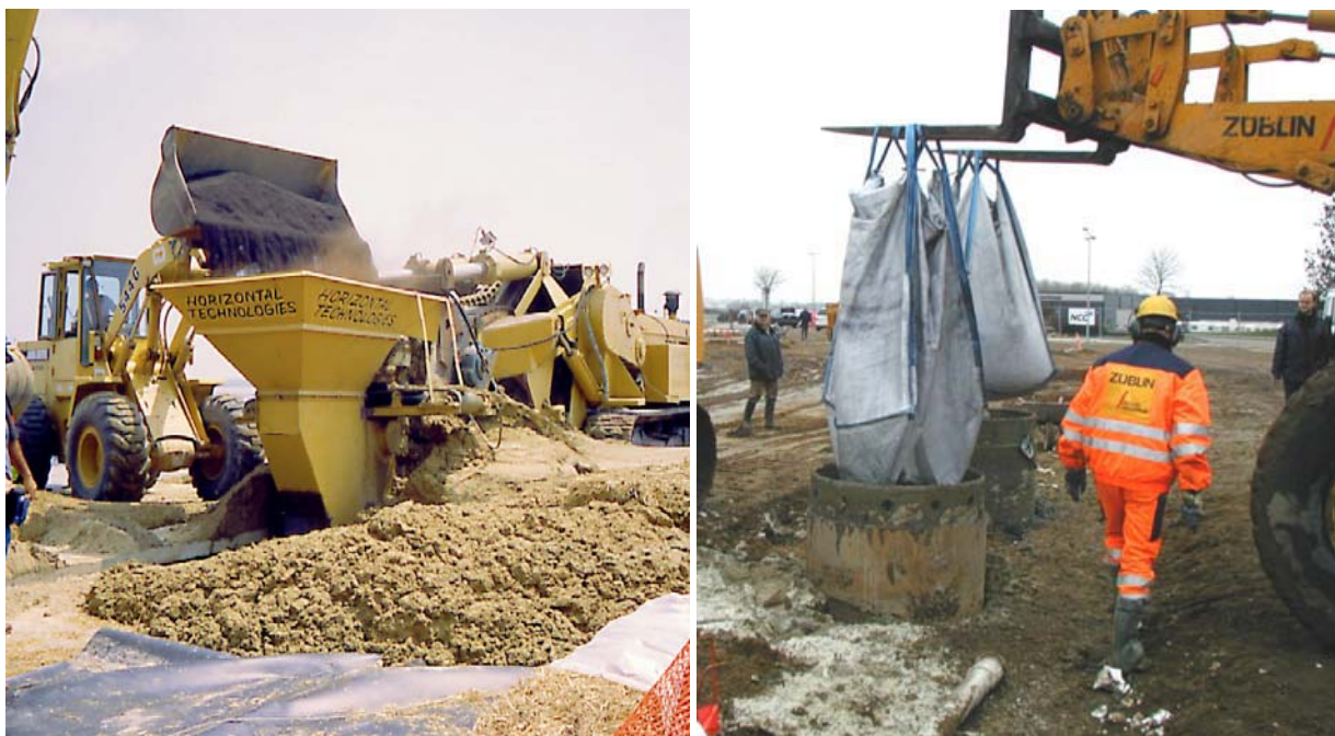
Figure E: Photos showing placement of materials into a PRB using on-site mixing of ZVI (left) and pre-mixed (right).
