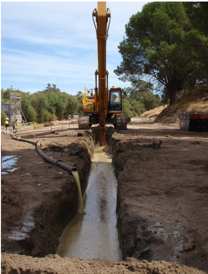
Installing the PRB (image courtesy Golder Associates)
