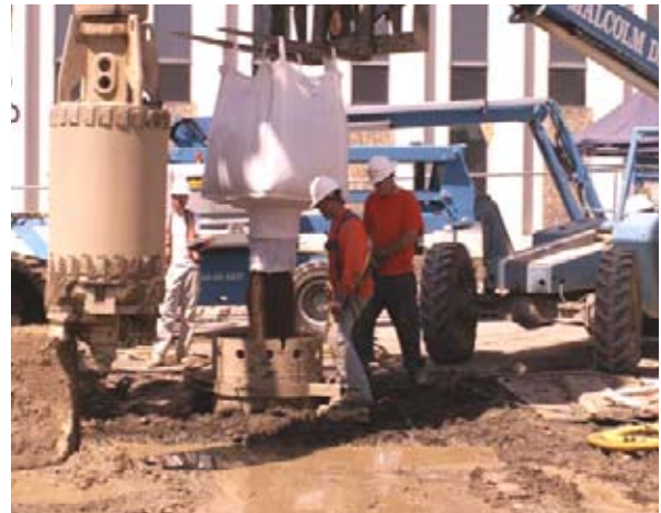
PRB construction with secant caisson and filling of caisson with iron/sand mixture.
