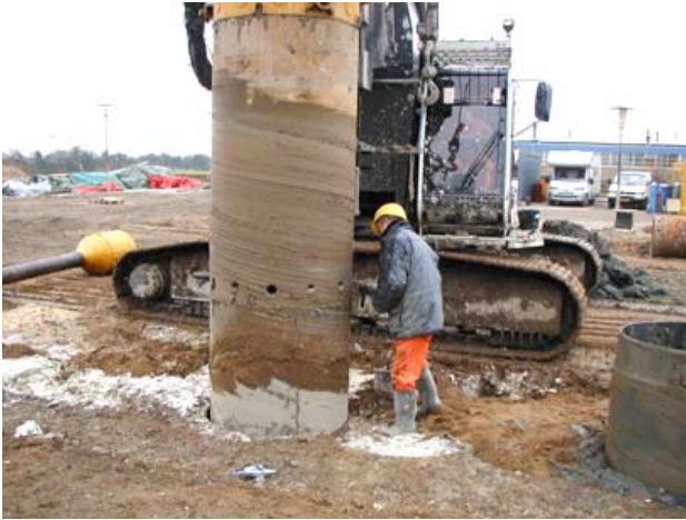
PRB construction with secant caisson and filling of caisson with iron/sand mixture.
