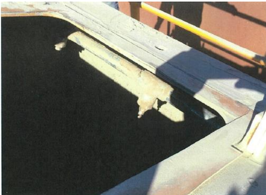
Plate 1: Dust suppression installed on the discharge head chute of a conveyor in the Crushing Plant
