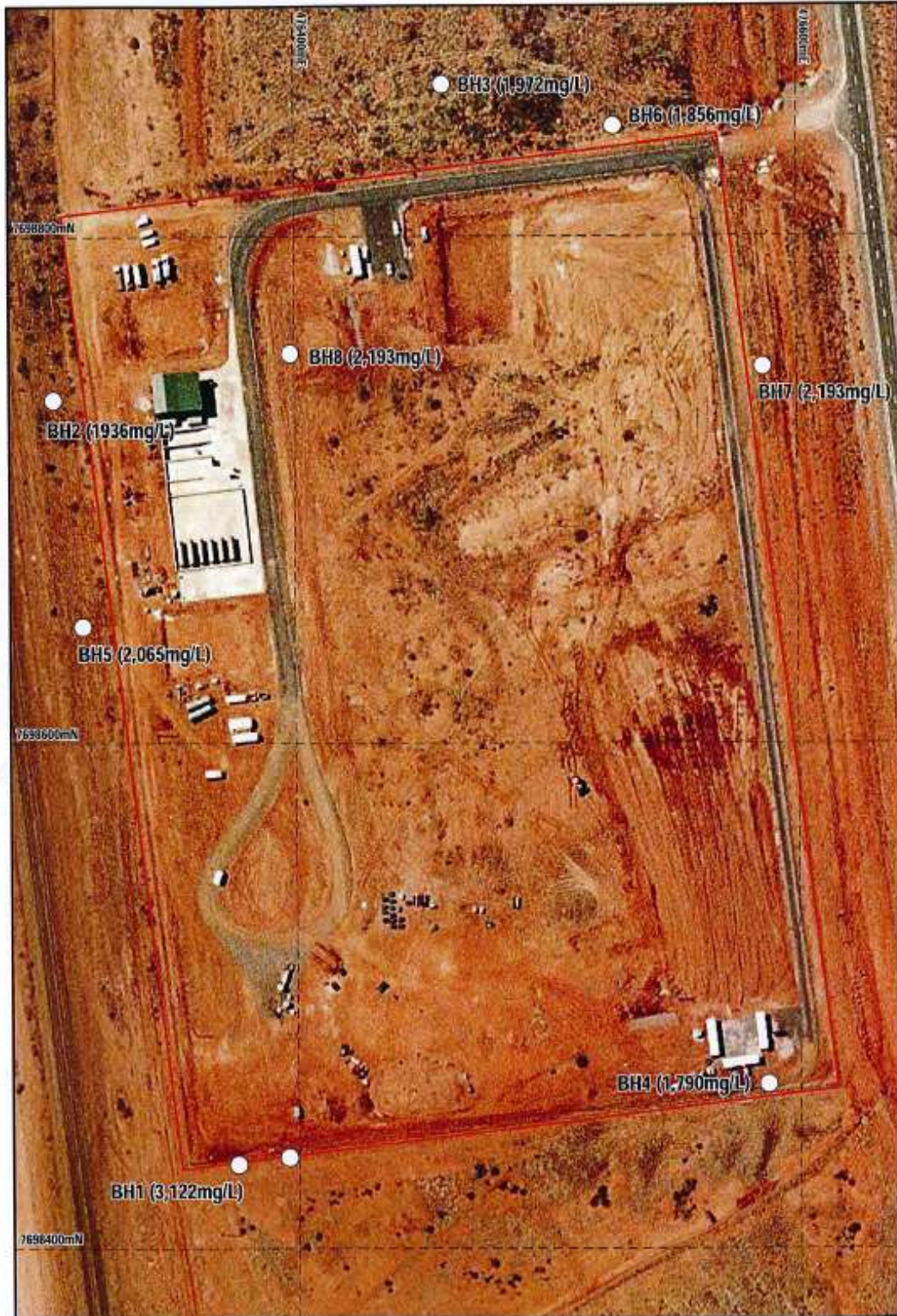
Figure 5: Groundwater monitoring bore location
