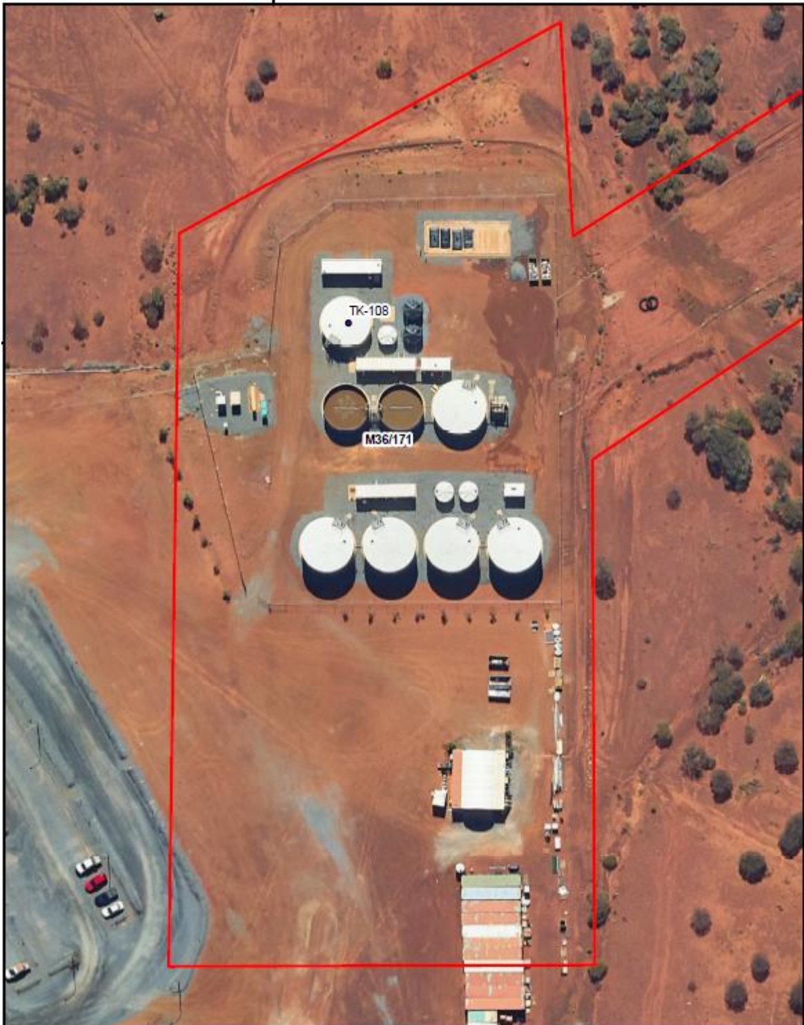
Figure 8: Irrigation tank TK-108 at Village WWTP
