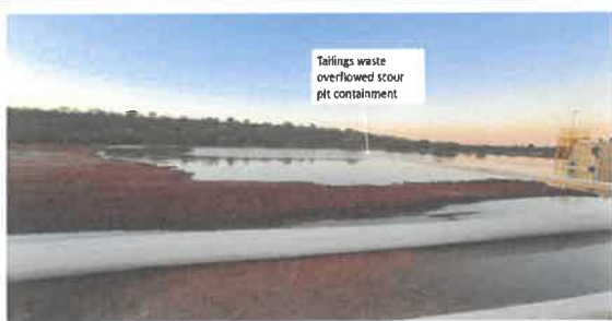
Figure 4. Photo of TSF2 pipeline spill showing waste overflowing scour pit
