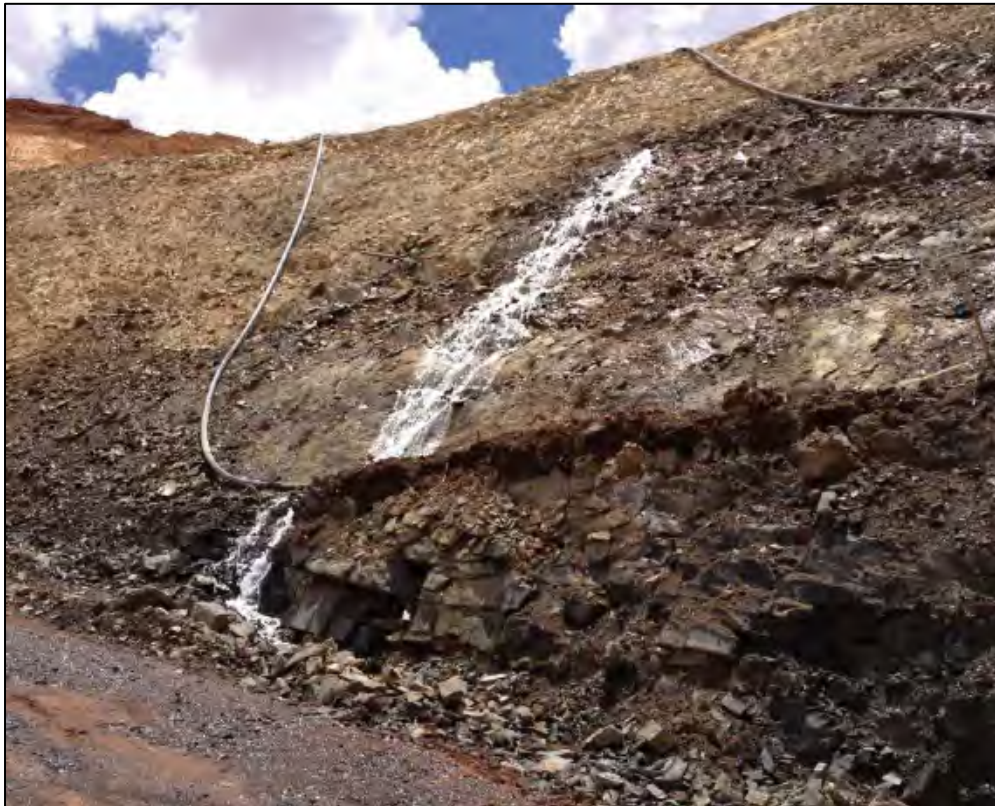
Figure 3.23: Major inflow location top of fresh rock around 345mRL (Ramelius 2014 Image 5)
