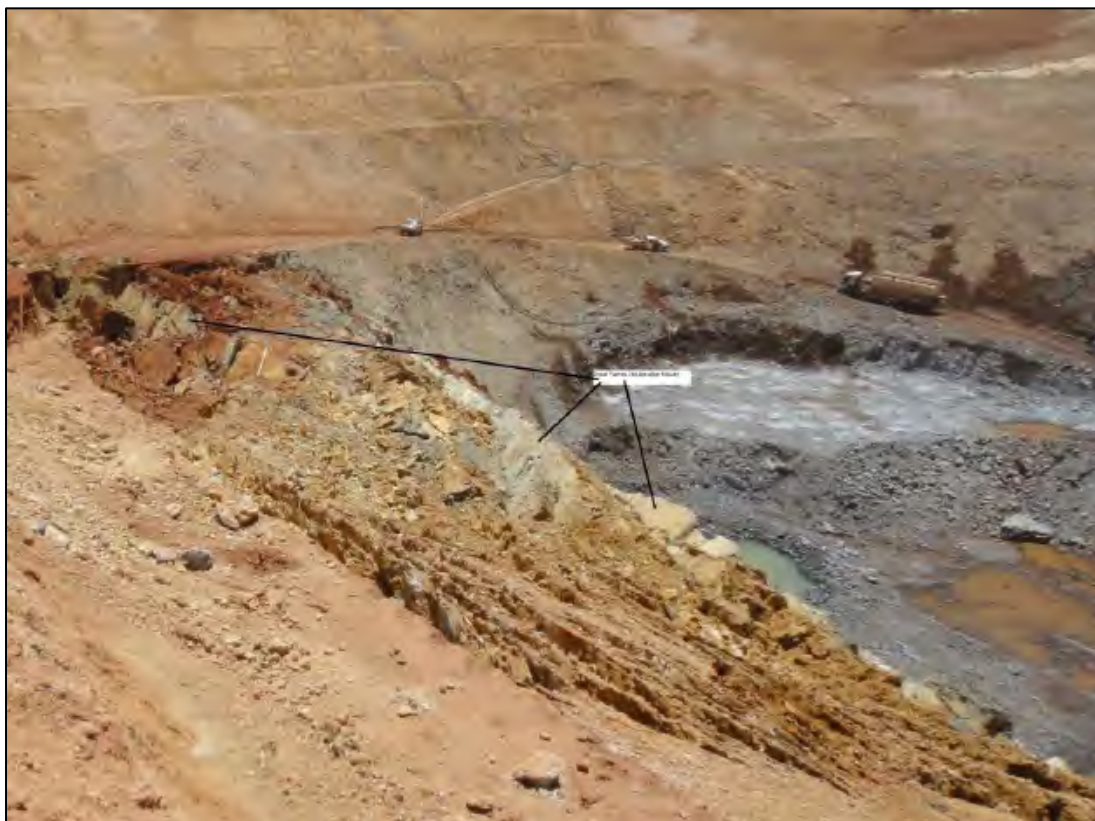
Figure 3.28: Top of Western wall collapse showing failure planes (Ramelius Image 8)
